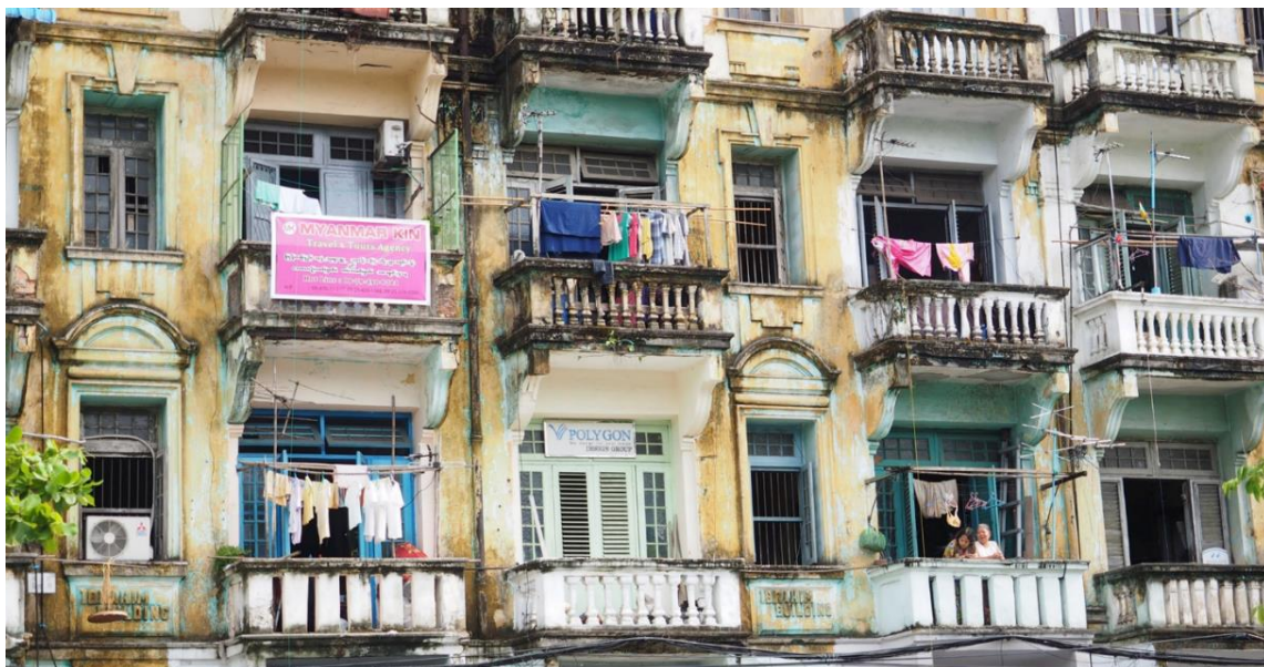
Figure 35 - Examples of unit by unit upgrading in Bogalayzay Street
