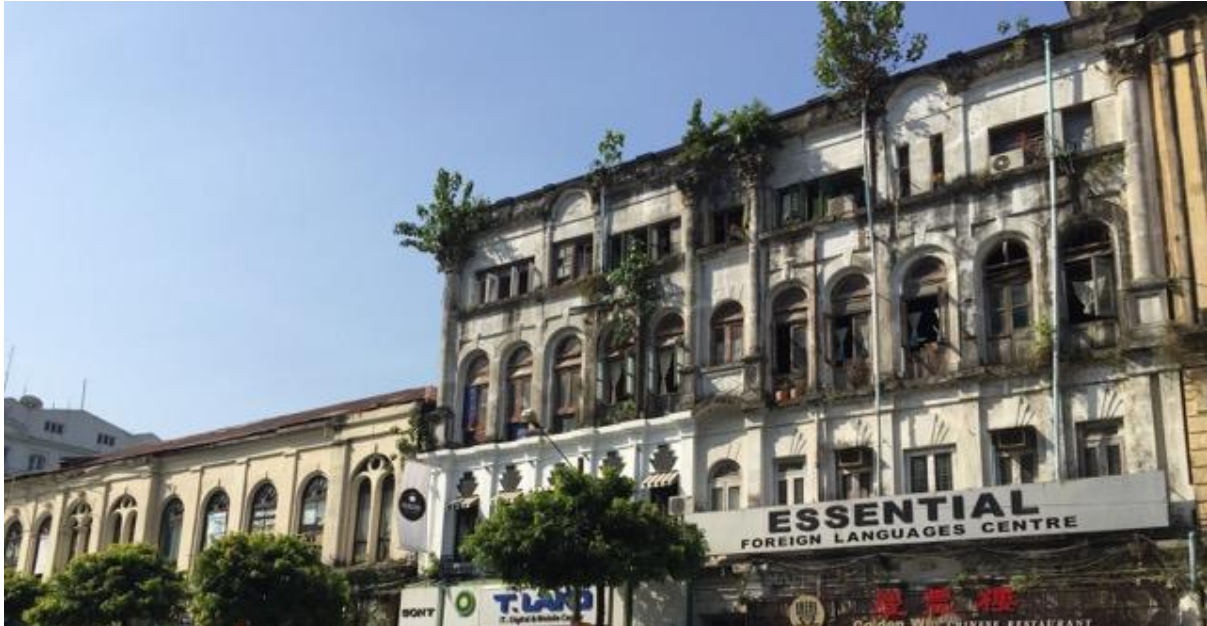
Figure 19 - The old and the new: freshly painted below banyan root infested facades
