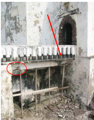
Entrance bridge supported by wooden beams to prevent collapsing
