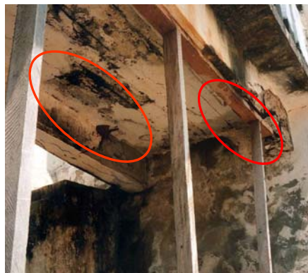
Entrance bridge supported by wooden beams to prevent collapsing
