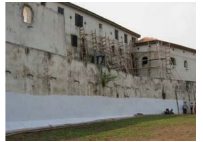
Terracing and landscaping works ongoing
